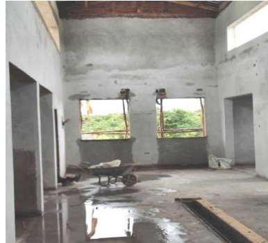
St. Peter's Hall construction.
