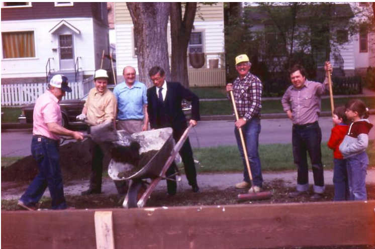
Laying the sod around the church building.
